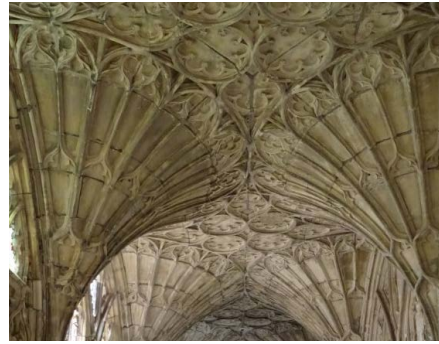
Fan vaulting, Gloucester Cathedral, by Philip Halling, CC BY-SA 2.0.
